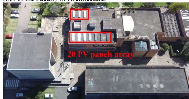
Figure 3: Actual PV solar panels with 7,7 kWp installed on the roof of the Faculty of Architecture.
