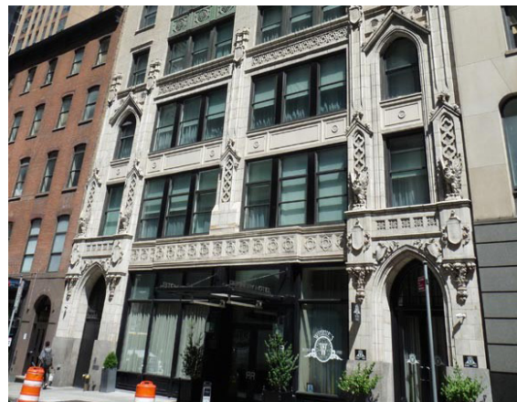
Fig 168. Luxury Hotel, New York. Fuente: Desconocido, 2020. Recuperado de: https://forgot-ten-ny.com/2020/10/38th-street-east-to-west/
