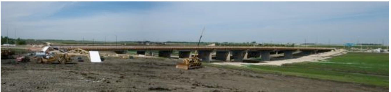
Floodway Bridge – Winnipeg, Manitoba
