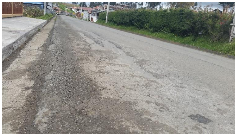
Figura 15: Falla Desnivel Carril – Berma, sector Déleg.
